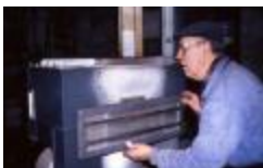
Herstel van mazoutkachel (Spanhove2013159)
